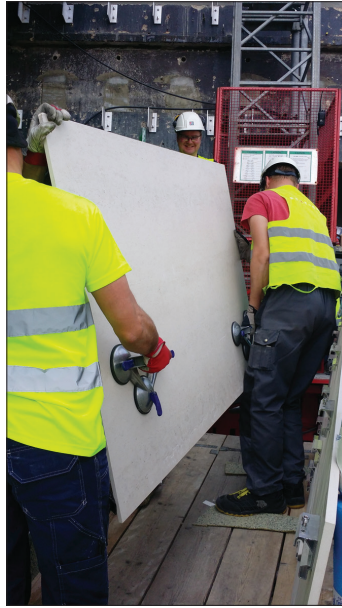
Figure 6a Manual handling of Dekton Panel for installation
