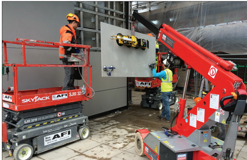
Figure 6b Installation of Dekton Panel with vacuum lifting device
